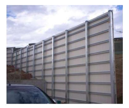
Where noise reduction up to 36 dB is required use a double D5 face wall -
